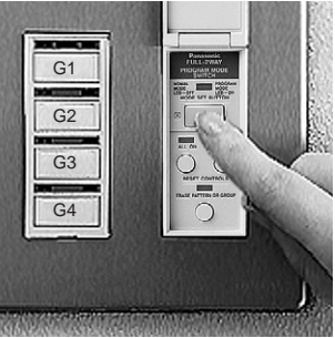
6 When group setting is complete, press the mode set button to change the system back to normal mode. (The Red LED will extinguish.)
