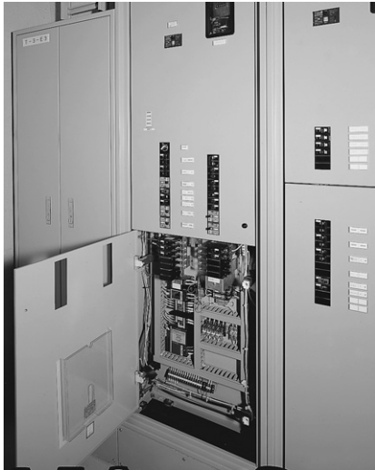
Inside Relay Control Panel
